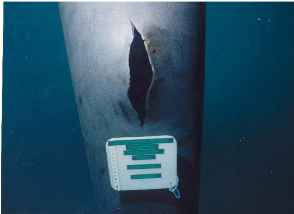
Figure 8 - Field Joint No. 301 from ZK 168
