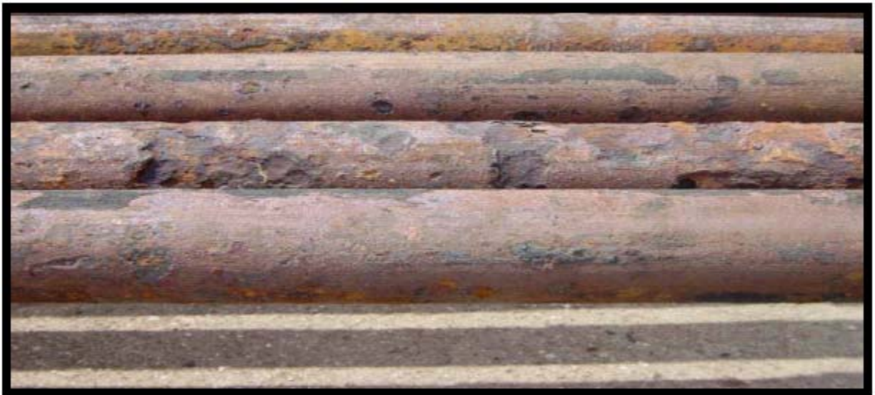
Figure 7 – Corroded Completion Recovered from ZK-144 Short String Against the Aquifer
