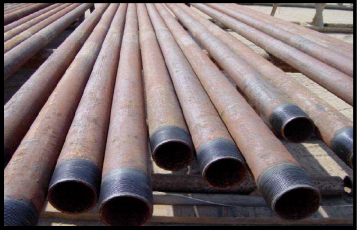
Figure 6 – Tubular Goods Recovered from ZK-234 after Twenty Years of Service
