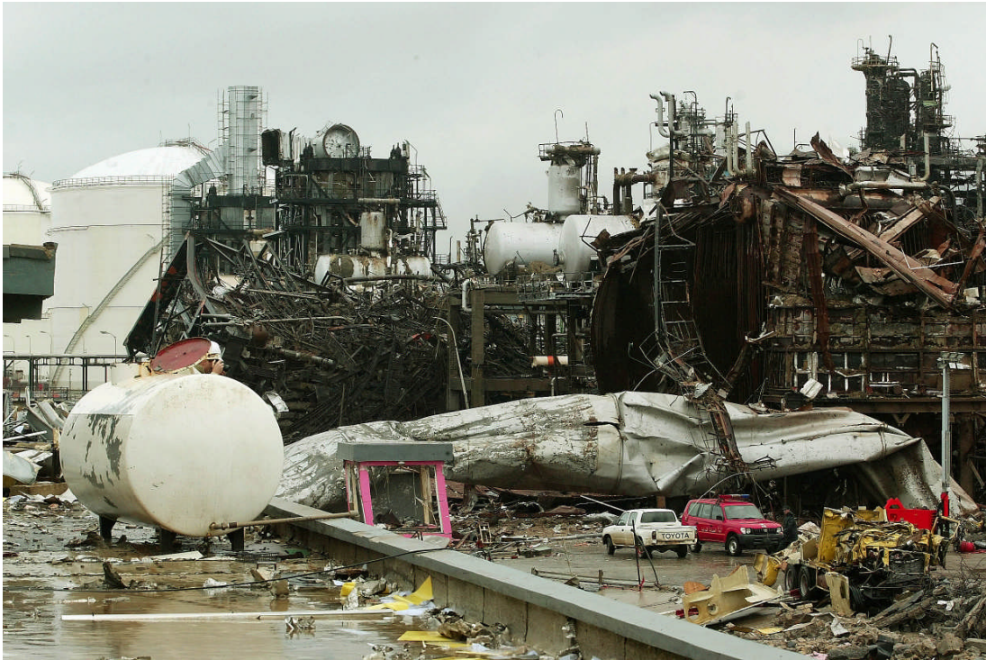
Figure 2: Failure in Safety Management
